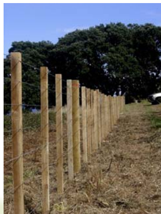
Newly built fence at Little Awanui
