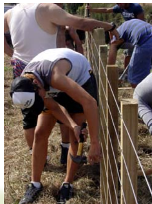
The whanau building the new fence
