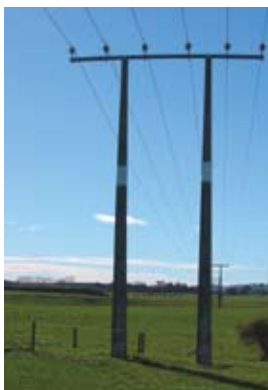
Pultron’s technology transforms fibre and resin into special lightweight materials that are strong and resistant to corrosion.
